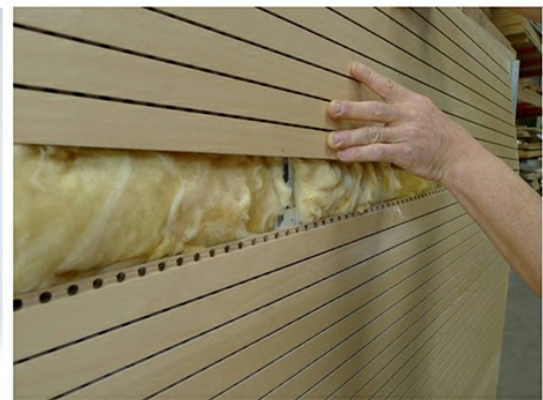
INSTALLATION: LIGHTWEIGHT STEEL KEEL SYSTEM
